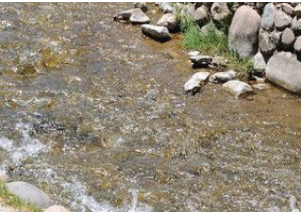
3m wide water channel. Base and sides incorporating stones / texture to create a natural character and generate water movement.
